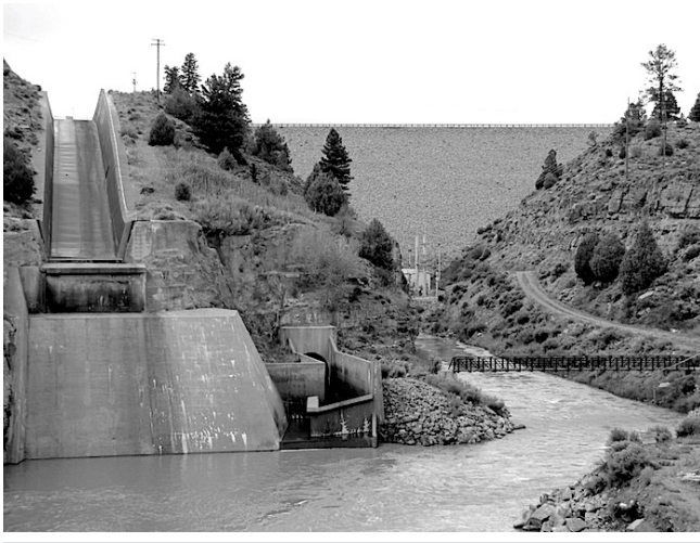
Fig. 3. A view of El Vado Dam and spillway looking upstream.
