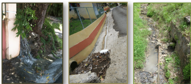
Fig. 9. Disposal of grey water generated from domestic activities. The pictures show grey water freely disposed through impervious structures and eventually reaching the environment. The photos were taken in areas of the upper portions of the Río Piedras Watershed.
